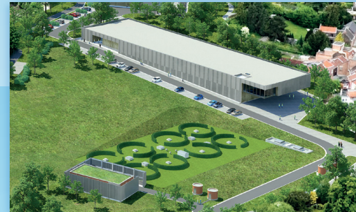
Drinking water treatment plant in Ans (Belgium) CILE - 35.000 m 3 /day
