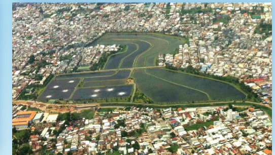
Wastewater treatment plant in Ho Chi Minh City (Vietnam) People's Committee of HCMC - 36.000 m 3 /day
