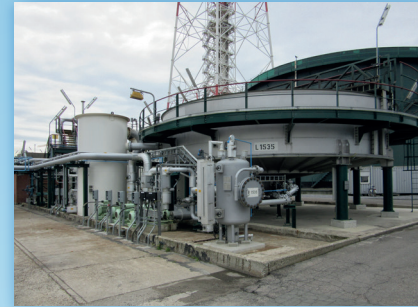
Process water treatment plant in Antwerpen (Belgium) - TOTAL - 7.200 m 3 /day
