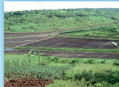
Irrigation of Kanyonyomba marshland (Rwanda) 63 km of canals spread over 6 km 2
