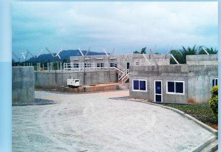
Drinking water treatment plant in Nsawman (Ghana) - GHANA WATER - 7.400 m 3 /day
